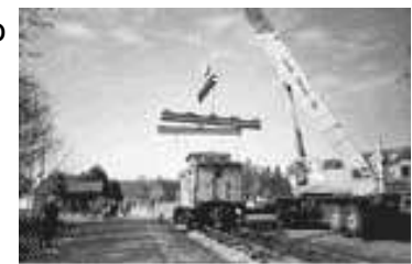
A crane was used to lower the caboose into position.
